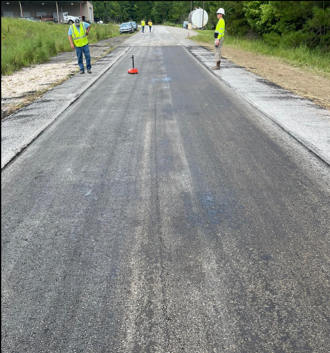
Initial compaction the day of paving
