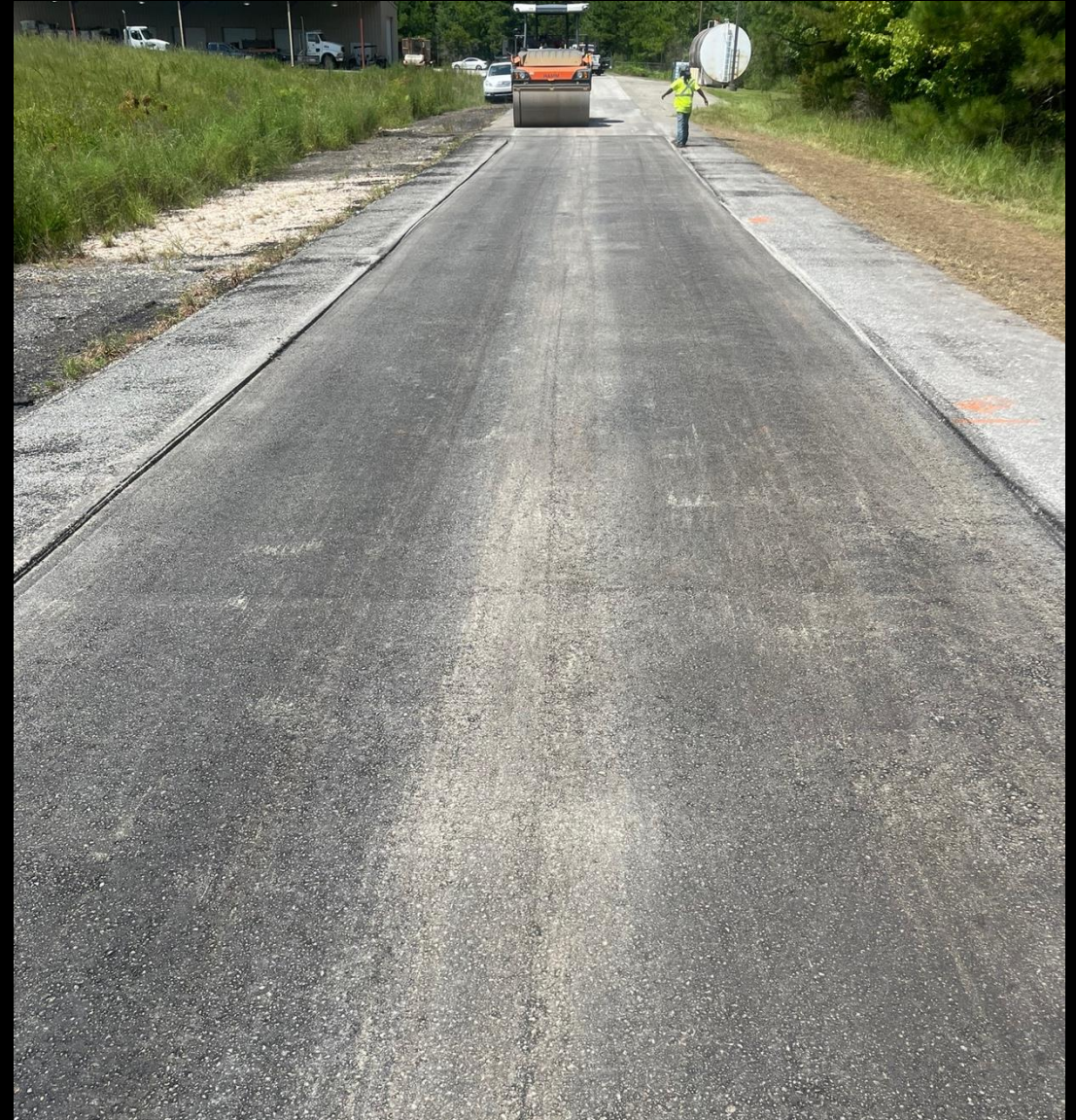
Secondary compaction the next day
