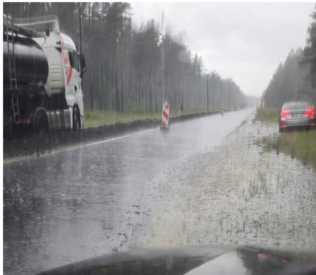
Insufficient drainage
