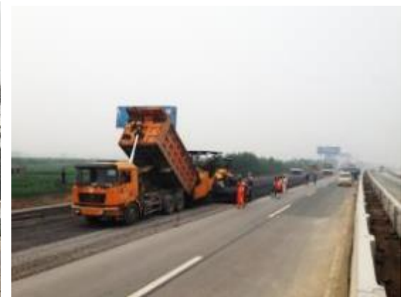
d) Paving with traditional equipment
