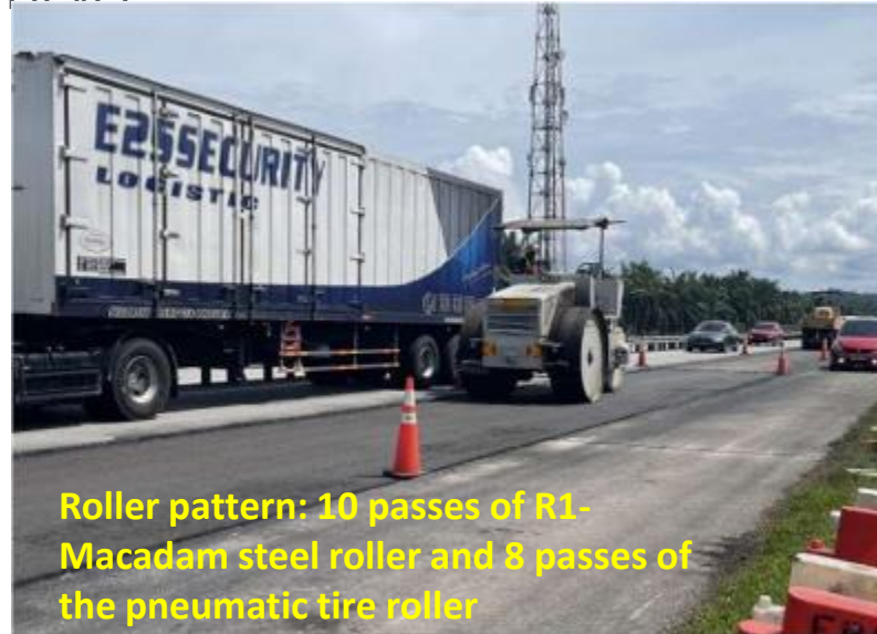
Paving of the emulsion CCPR mixture
