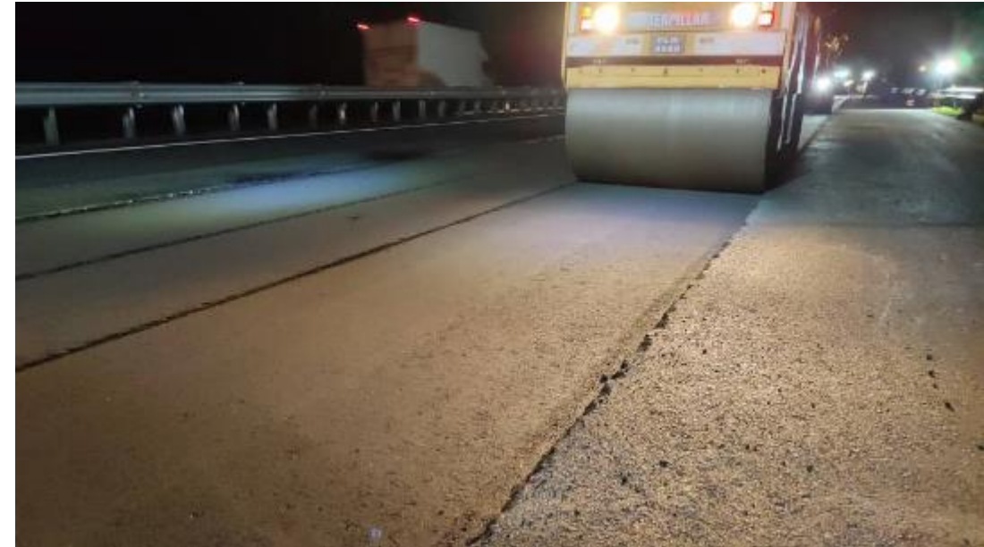
October 18, 2024 paving of the emulsion CCPR at night
