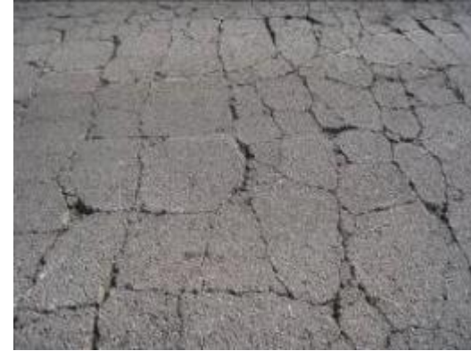
Distressed Asphalt Concrete
