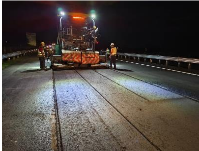
October 18, 2024 paving of the emulsion CCPR at night
